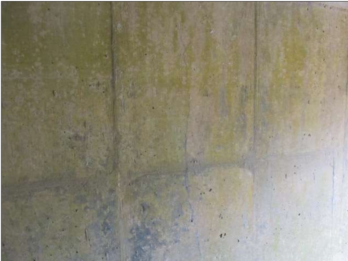
H/L VERTICAL CRACKING ALONG THE INT. AND EXTERIOR WALLS.
